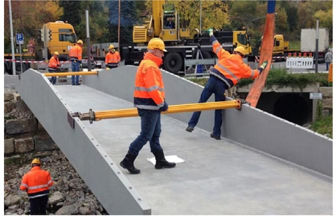
Bridge made of carbon concrete composite
